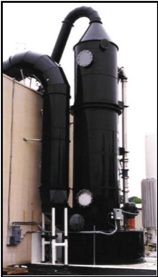
10,000 ACFM Dakota Scrubber™ removing triethylamine (TEA) emissions from phenolic urethane cold box process
