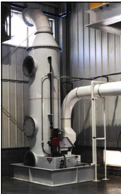
4,300 ACFM Dakota Scrubber™ con polypropylene safety dam
